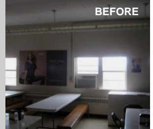
Junior High: Replaced existing aluminum single pane windows with new aluminum thermally broken, double pane insulated unit. Restored to original window opening.
