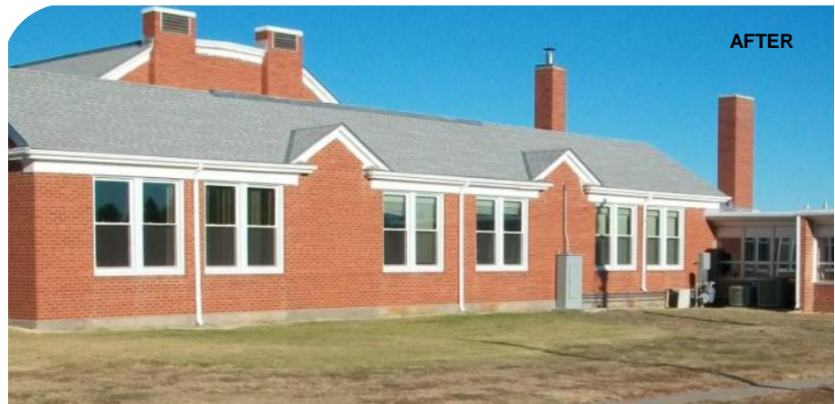
Damar Junior High: Replaced old single pane windows with new vinyl thermally broken double pane insulated units. Removed old window AC units and antiquated boiler system and installed efficient HVAC system for improved comfort and indoor air quality.
