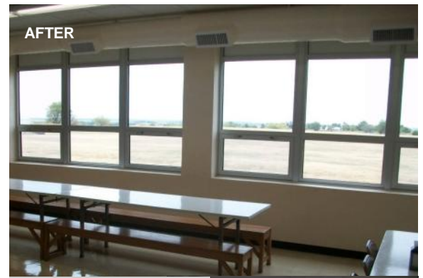
Junior High: Replaced existing aluminum single pane windows with new aluminum thermally broken, double pane insulated unit. Restored to original window opening.
