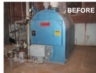
High School: Replaced the burner on the existing boiler with a new high efficiency unit.
