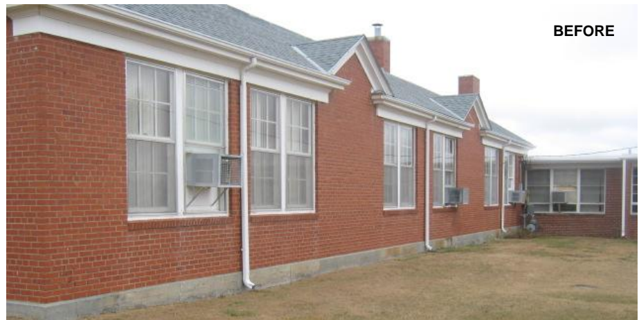
Damar Junior High: Replaced old single pane windows with new vinyl thermally broken double pane insulated units. Removed old window AC units and antiquated boiler system and installed efficient HVAC system for improved comfort and indoor air quality.
