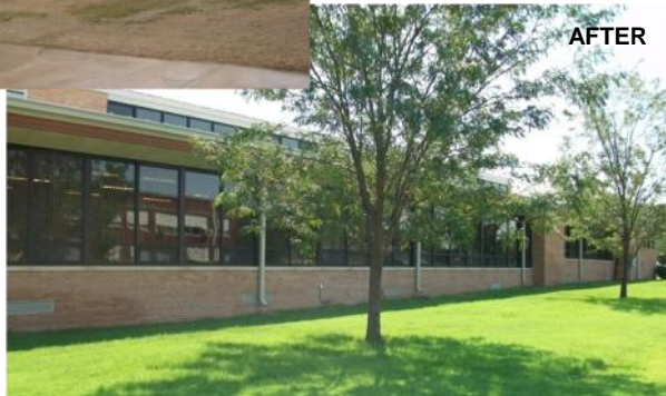
High School: Replaced single pane steel windows with new aluminum thermally broken, double pane insulated units with tinted glass. Replaced original 1954 steam unit ventilators and window AC units with new steam/chilled water unit ventilators.
