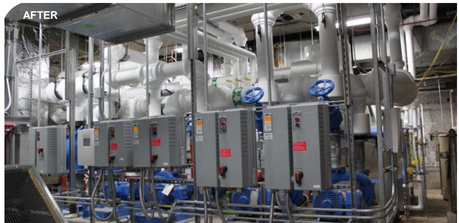
Administration Building North Mechanical Room: Replaced old air handling units with new Water Source Heat Pumps (WSHP) tied to a hybrid WSHP loop combining new geothermal wells, existing equipment and new high efficiency supplemental hot water boilers.
