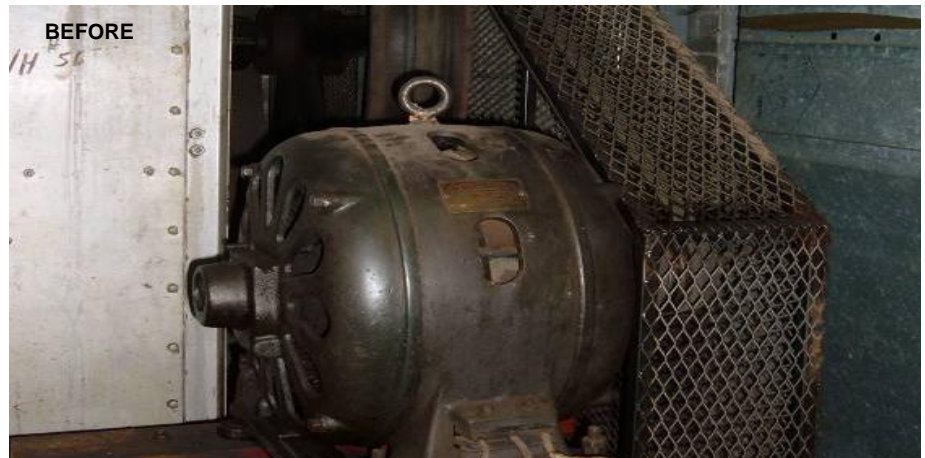
Administration Building North Mechanical Room: Replaced old air handling units with new Water Source Heat Pumps (WSHP) tied to a hybrid WSHP loop combining new geothermal wells, existing equipment and new high efficiency supplemental hot water boilers.
