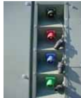
Figure 5. Cam-type connectors with and without cables connected
