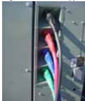
Figure 5. Cam-type connectors with and without cables connected
