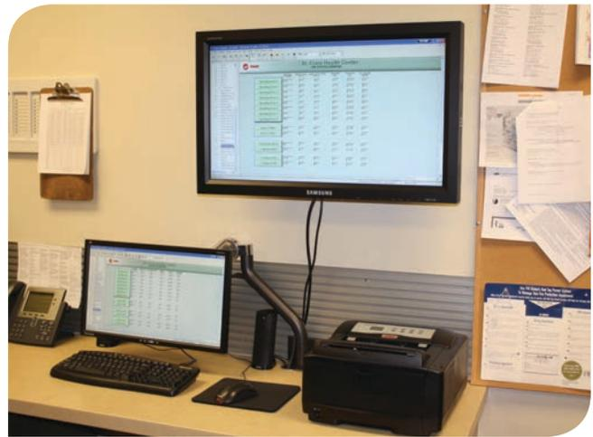
A BAS with custom dashboards displays current conditions and energy use to ensure efficiency.
