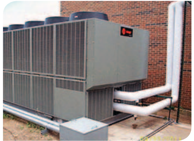
A Trane high-efficiency air-cooled rotary chiller helps to reduce Rock Creek Unified School District's energy costs.
