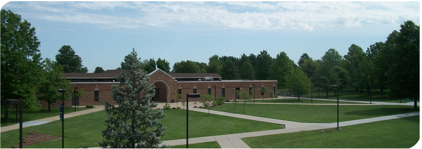
Pictured Above: The William C. Hopkins Student Services Center received high efficiency lighting upgrades, high efficiency water conservation fixture upgrades, a new building control system and energy efficient HVAC upgrades.
