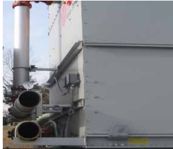
Figure 6. 270 ton CT piping detail
