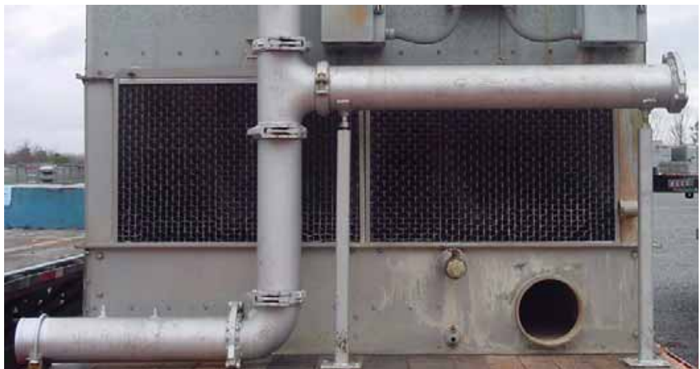
Figure 7. Inlet piping and (1) 10 in. outlet on back of tower (500F0AC & AH only)
